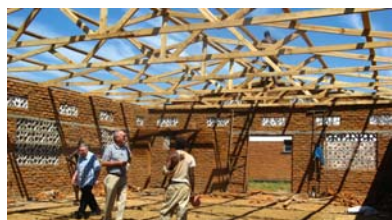
Roof open, with Fr. Owen inspecting the work.
