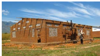
Nearly completed Hall
